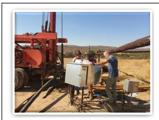
The mechanical pump in the Waterberg borehole stripped almost two months ago and caused serious damage to the rods and to the pump. It took a concerted effort to remove the damaged pump which has now being replaced with a submersible pump. The borehole was back in service before month end and once again delivering up to 300,000 liters per day into the irrigation dam.
